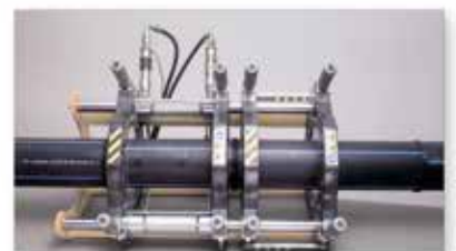
Stage 5 welding with element in pressure
