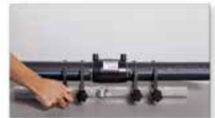
Clamps pipe and align it.
