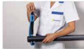
Cut the pipe with the pipe cutter.
