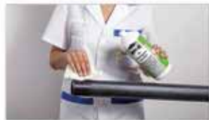
Clean the surfaces with a suitable detergent.
