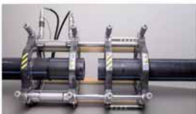
Place the elements to be welded into the machine.
